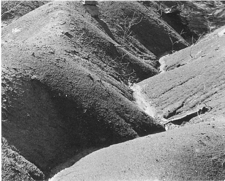
V-shaped gullies in a material relatively high in clay.
